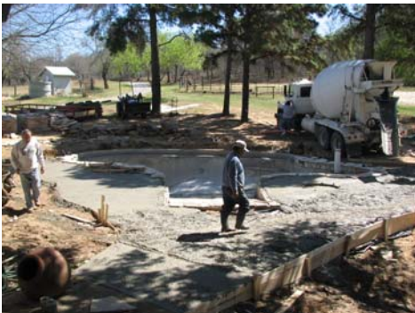
Decking, Tile, Coping
