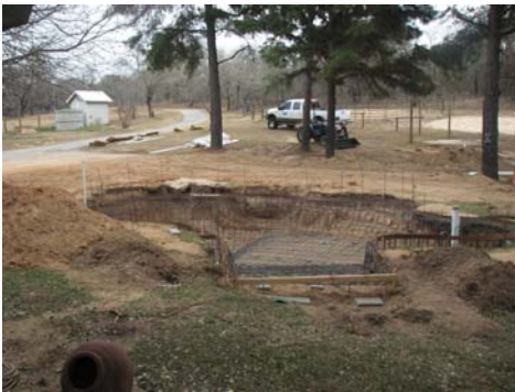
Steel & Plumbing rough-out
